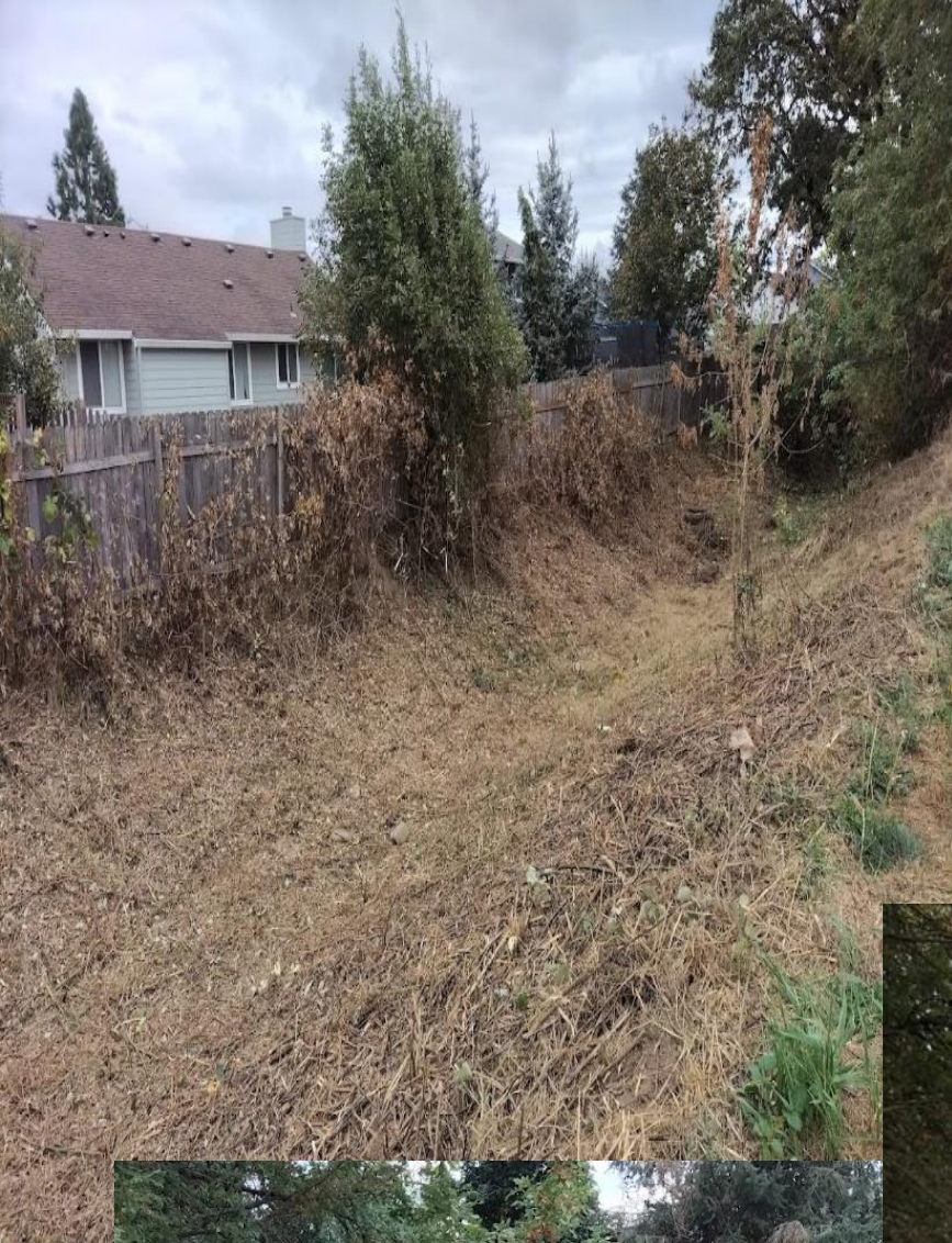
Public Works Maintenance Crews Removing Bush in a Storm Swale to Help Alleviate the Possible Flooding issues in Big
