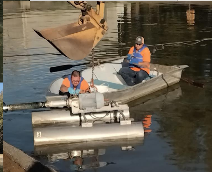
Waste Water Crews Removing Aerators from Aeration Basin.
