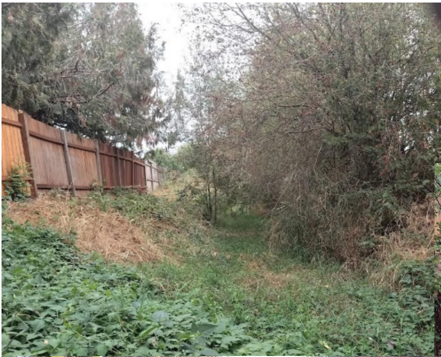
Utility Crew Hand Dug the Channel Out of Storm Ditch
