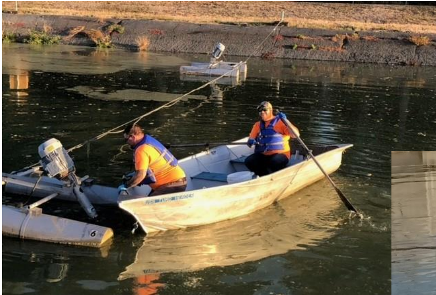
Waste Water Crews Removing Aerators from Aeration Basin.
