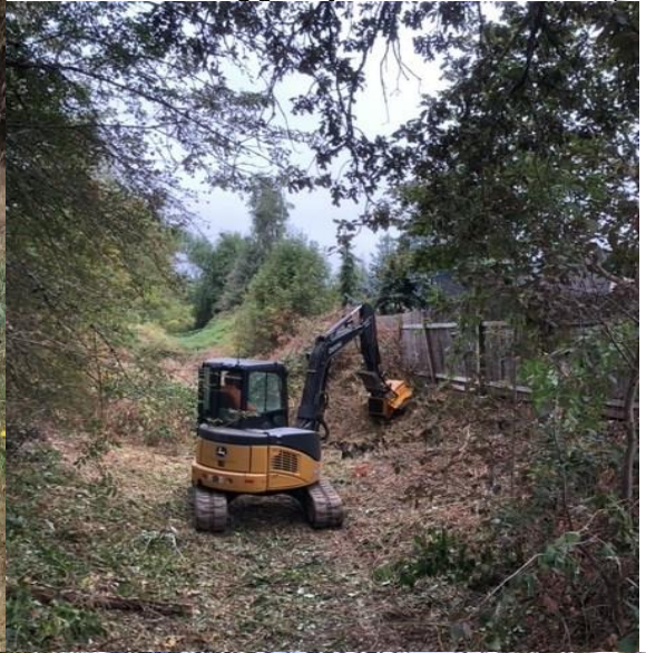
Public Works Maintenance Crews Removing Bush in a Storm Swale to Help Alleviate the Possible Flooding issues in Big
