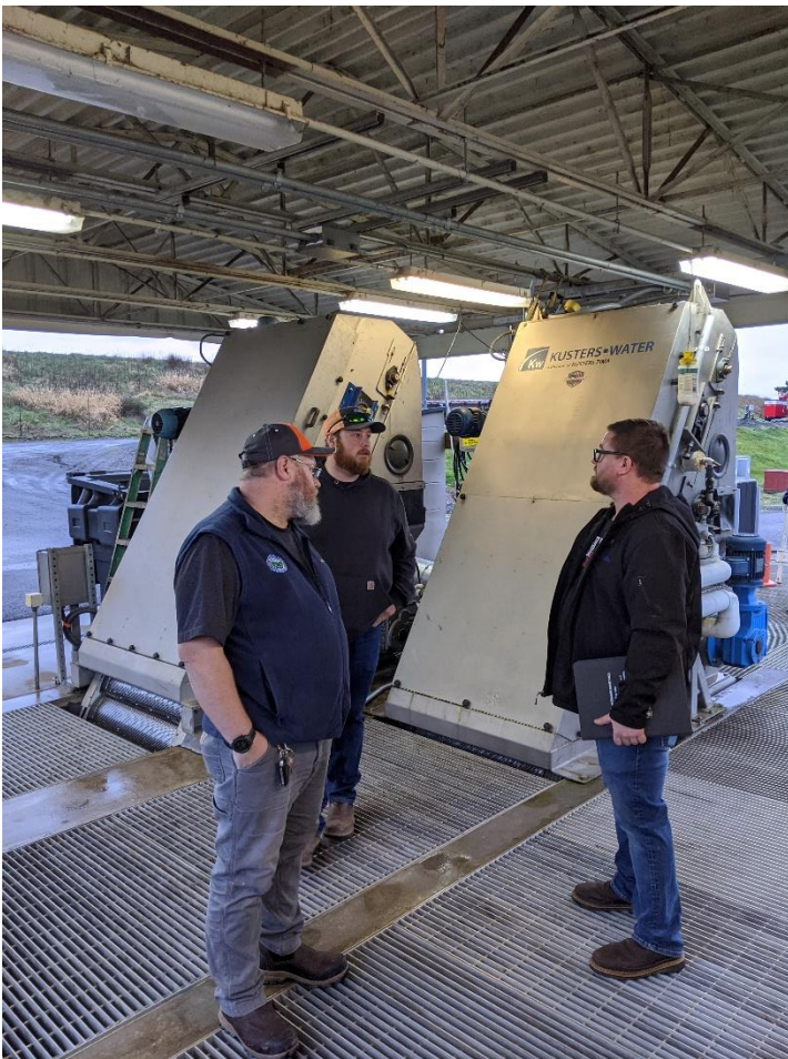
Top: Wyatt Kylo grading West Lane. Left: Assistant Waste Water Plant Operators James Clifton and Mitch Jaspers meeting with New Plant Lead Operator Seth Kelly
