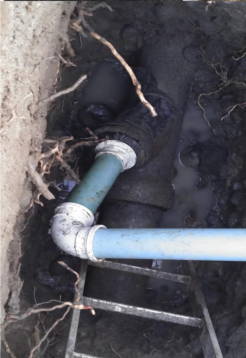
Public Works Crews replacing a failed sewer lateral that was filled with tree roots.
