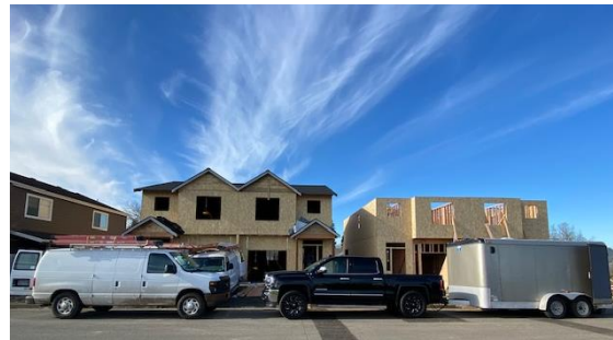
February 9, 2021: 2 New Duplex's under construction on Eckard Dr.
