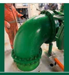
The gasket inside the flange failed and leaked.
