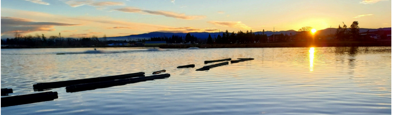
City of Molalla Wastewater Treatment Center
