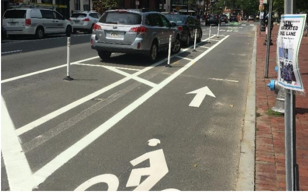
Example of One-way Parking Protected Bike Lane
