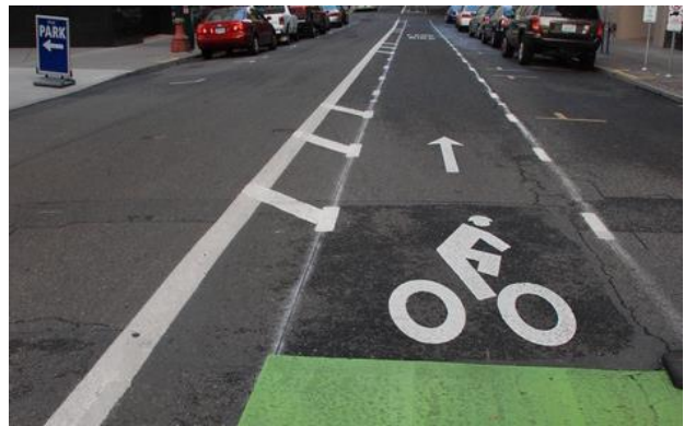
Example of Buffered Bike Lane
