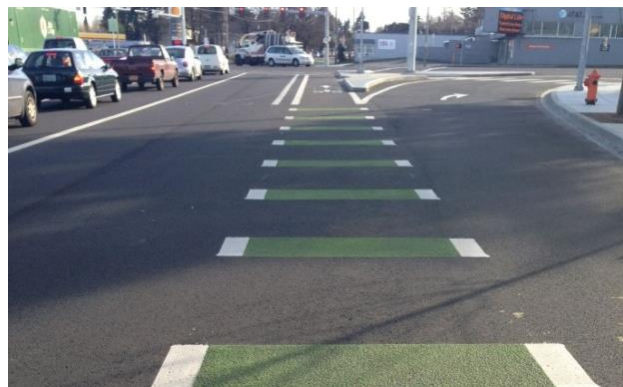
Example of Pavement Markings Through Intersection
