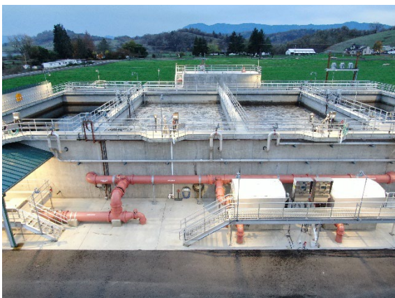
An example of the SBR type Wastewater Treatment Plant that will be built in Molalla, in part with Sewer SDC's
