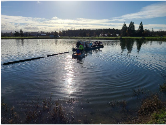
These Lagoons have served for the City's needs for many years, but population now exceeds their capacity. A new Plant is in Design.
