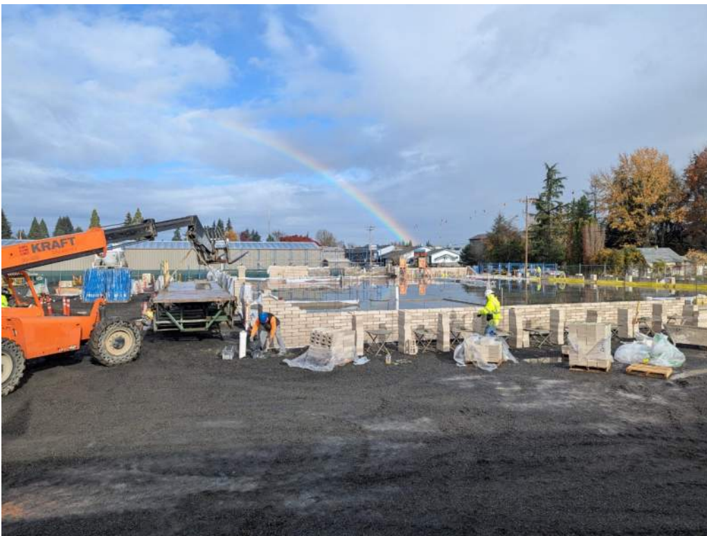
Figure 4- 11.21.2024- Masonry wall installation with rainbow
