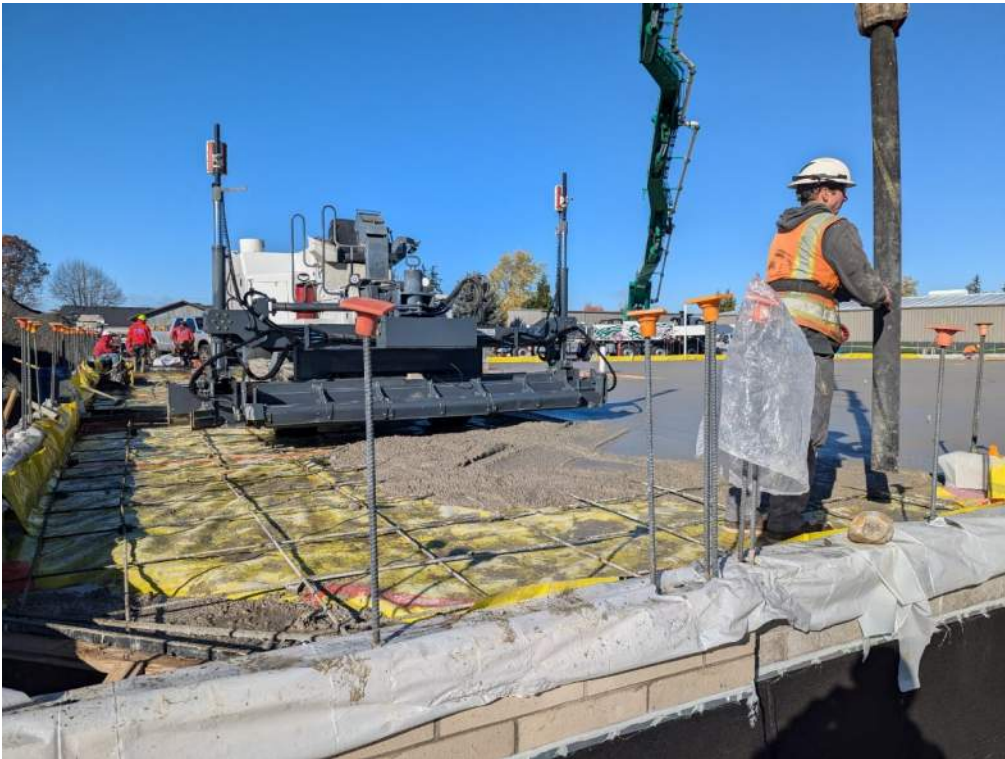
Figure 8- 11.6.2024- pouring concrete slab entry zone
