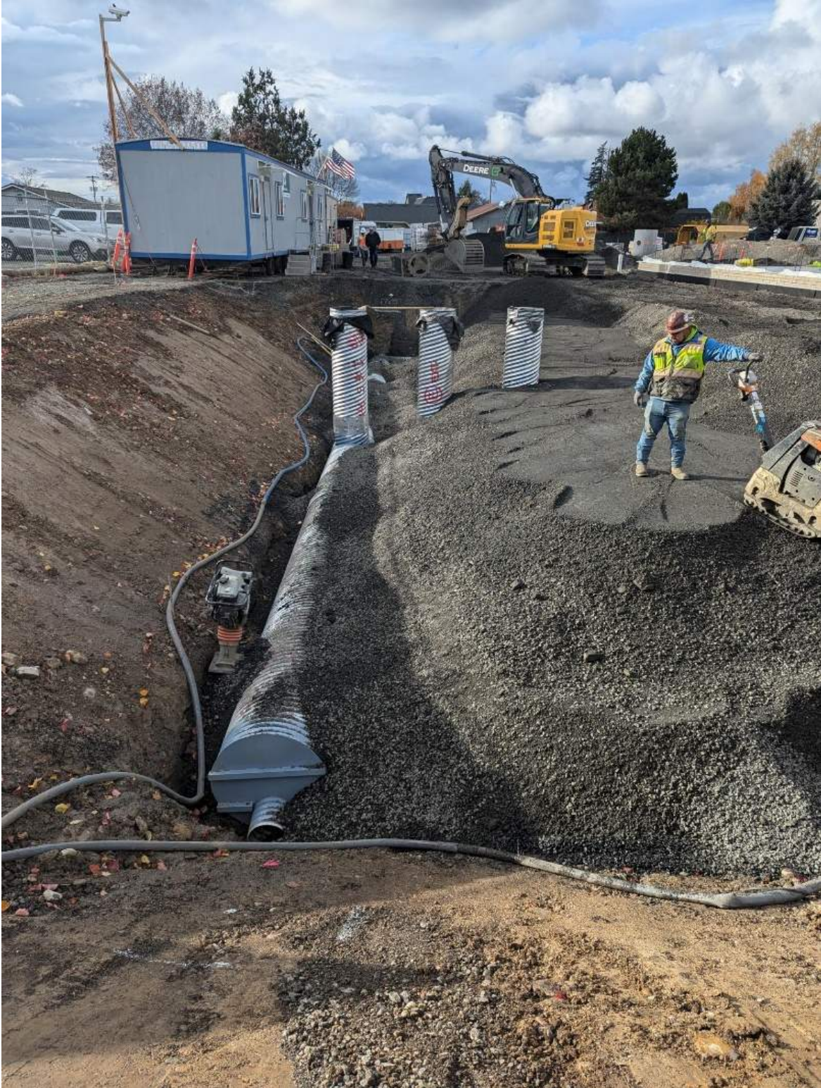
Figure 6- 11.14.2024- New underground storm system installed
