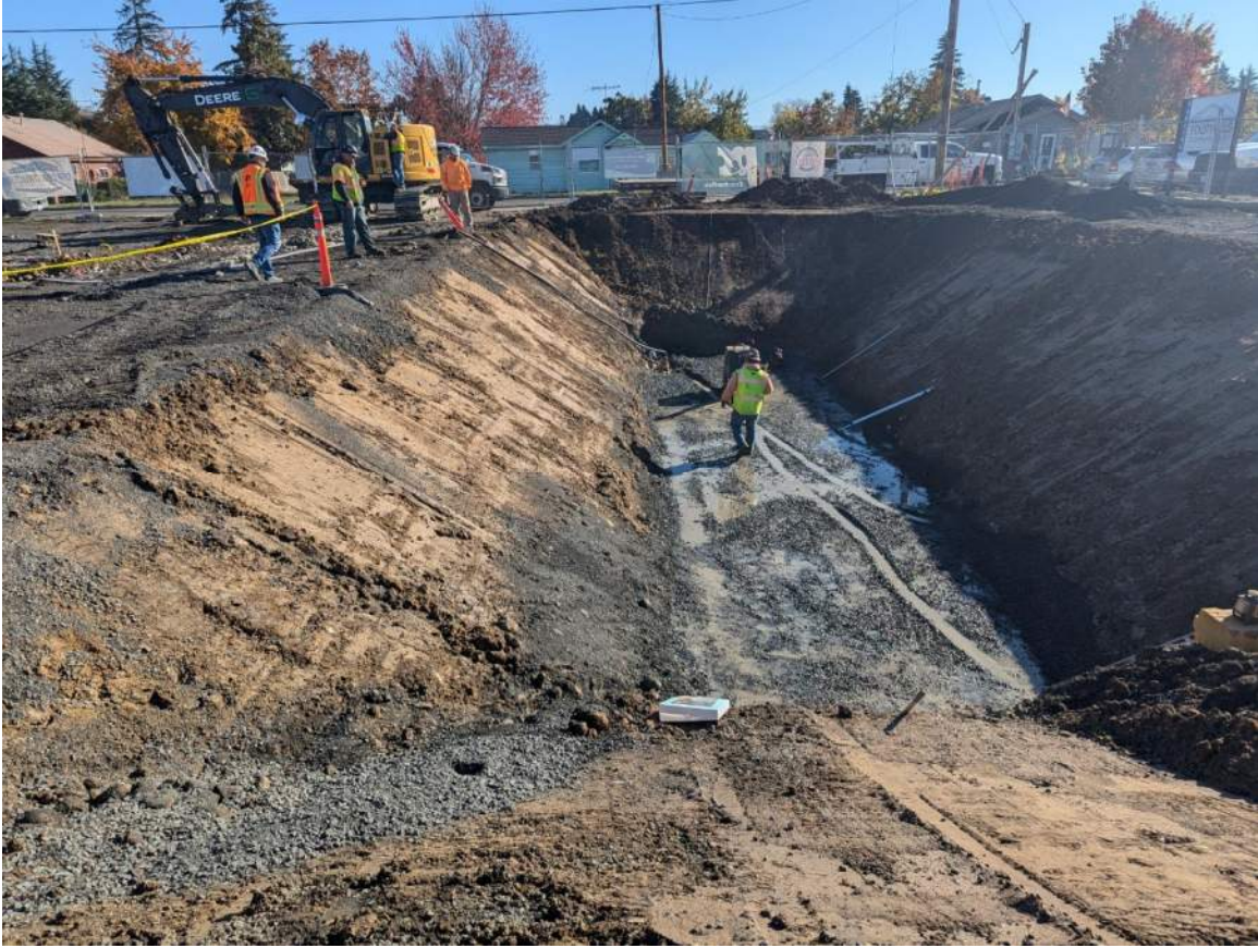
Figure 5- 11.6.2024- Big hole in ground for new storm detention system
