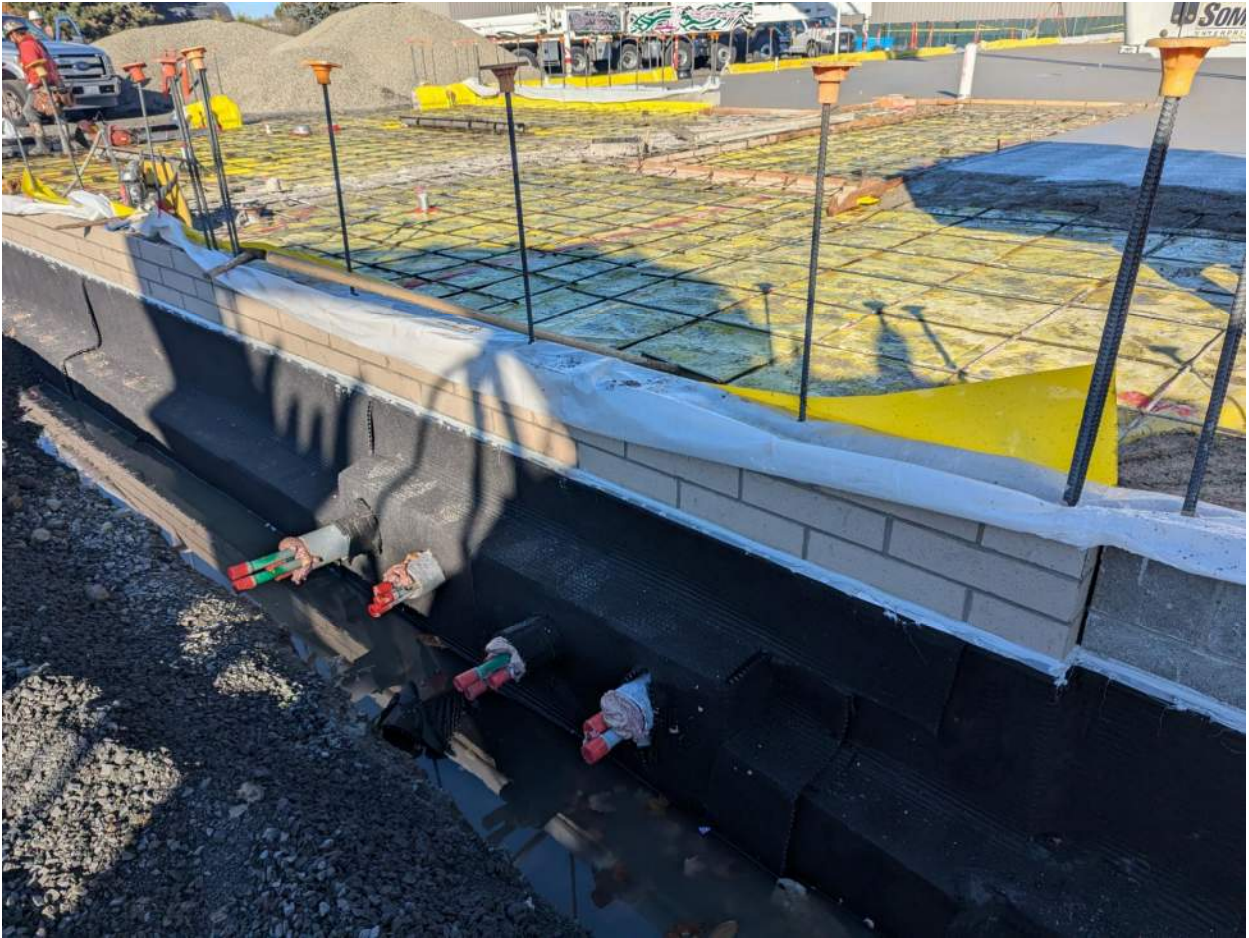
Figure 9- Concrete slab pour, below grade waterproofing of utility penetrations
