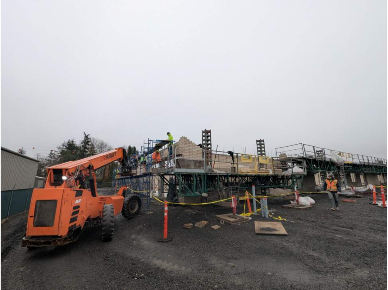
Figure 2- 12.12.2024- Masonry wall installation, scaffolding
