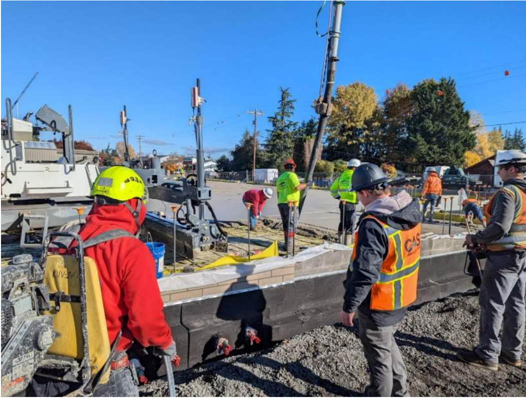
Figure 7- 11.6.2024- Pouring concrete slab
